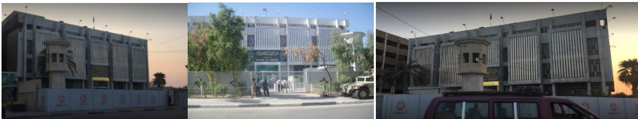
Figure (10): shows the external form of the Central Bank of Iraq, Basra branch, Source: https://cbi.ia/news/view/499
